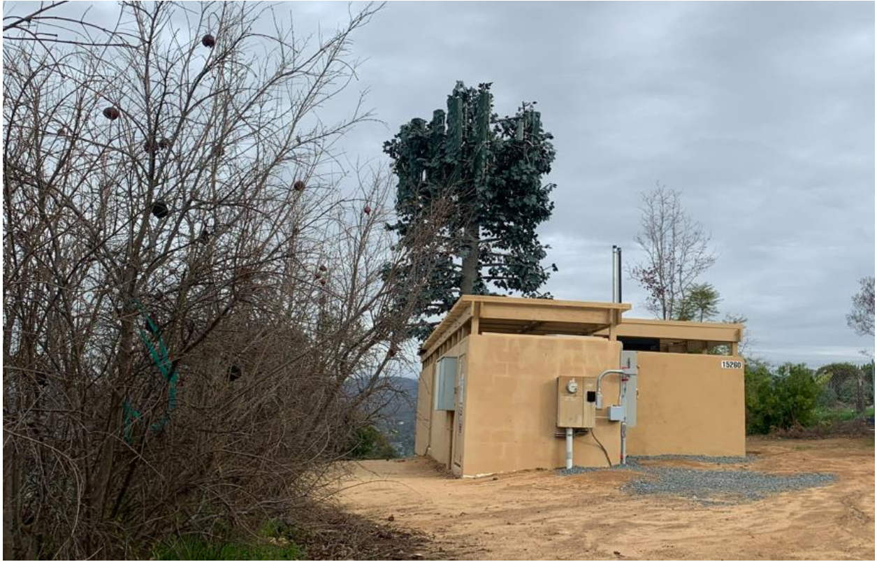
View North at Site
