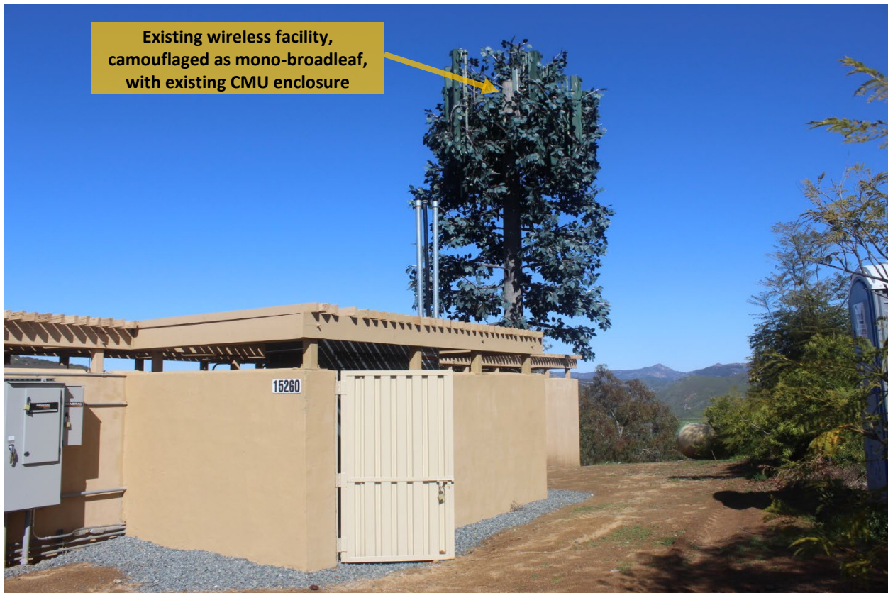
Figure 1: Existing 36.9-foot-tall wireless facility and 432 feet CMU equipment enclosure.
