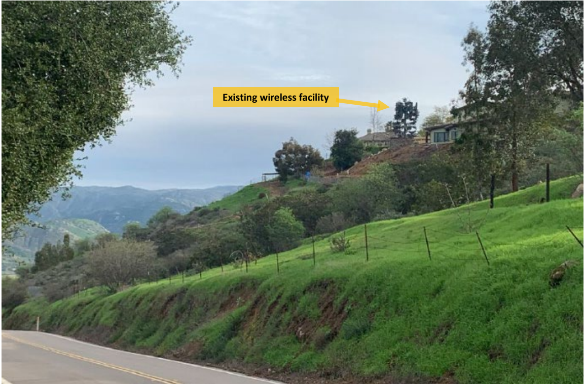
Figure 2: Existing 36.9-foot-tall mono-broadleaf wireless facility looking east toward the site from Bandy Canyon Road.
