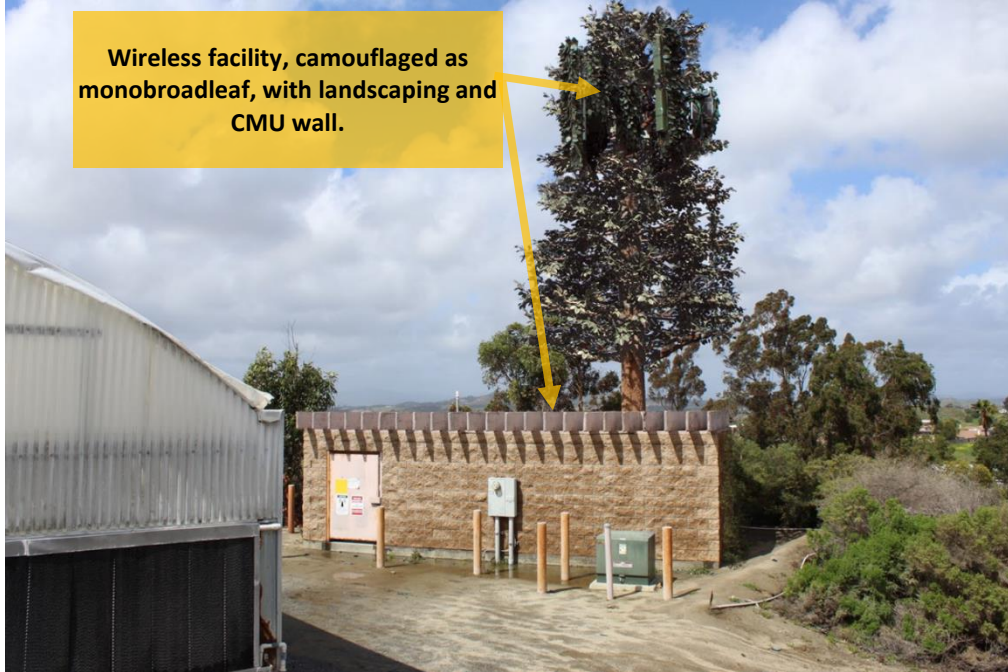
Figure 1: Existing 40-foot-tall wireless facility camouflaged as monobroadleaf, on the site of an existing nursery, looking North toward site.
