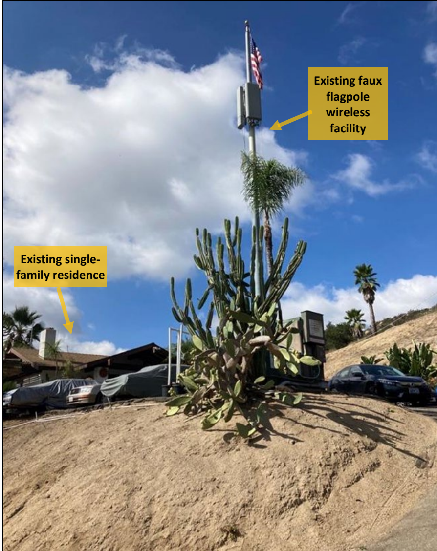
Figure 1: Existing 42-foot-tall faux flagpole wireless facility near the single-family residence looking from the existing driveway.
