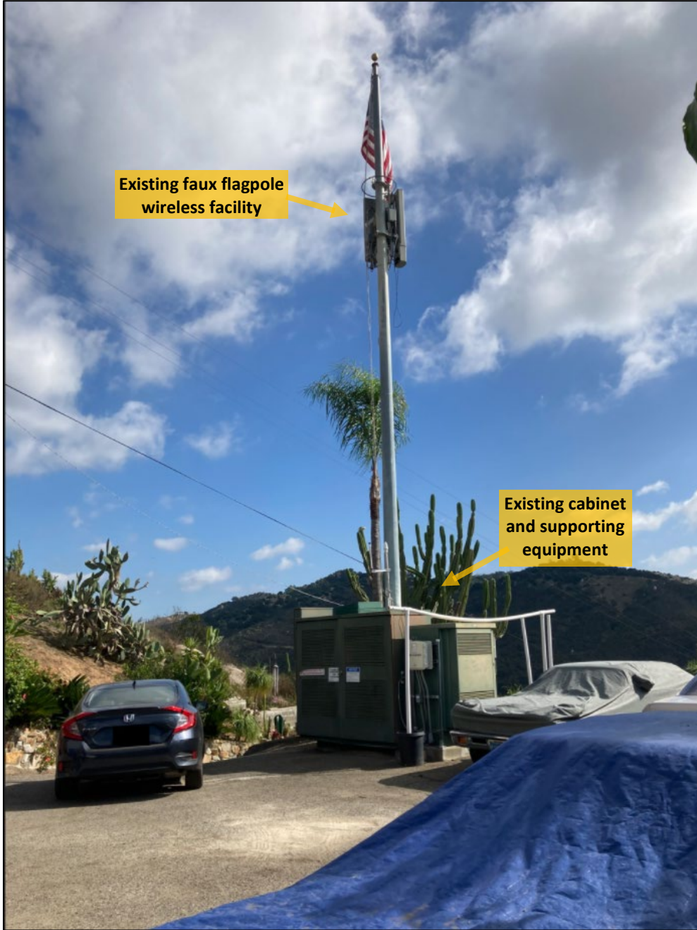
Figure 2: Existing 42-foot-tall faux flagpole wireless facility looking from the existing single-family residence.
