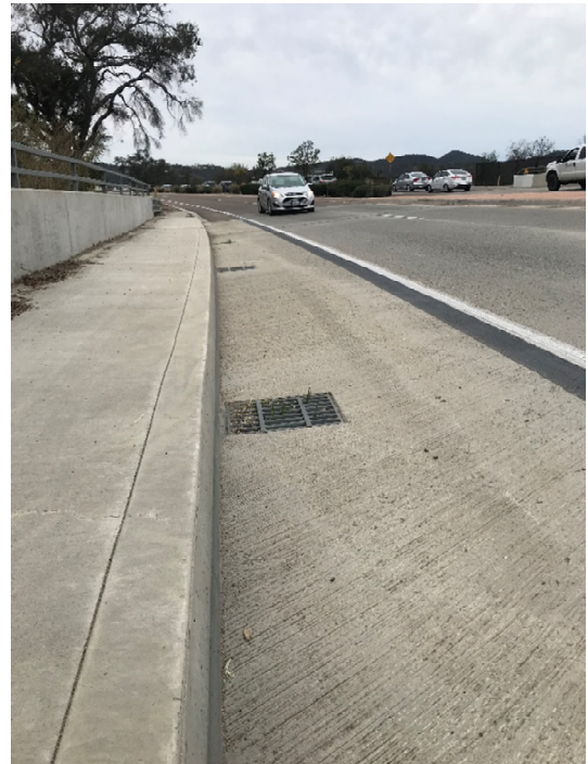
Figure 20: Class II bike lane with drainage inlet.
