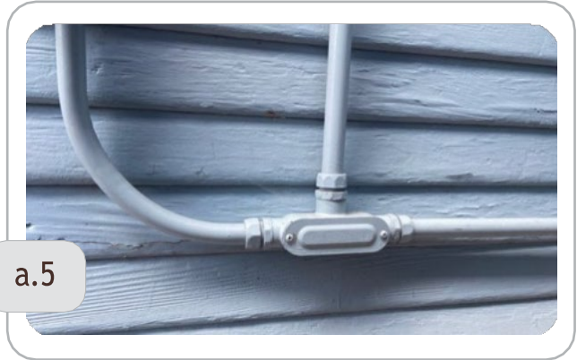
Surface mounted utility conduit
