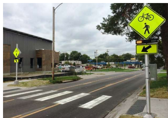
Figure 13: Activated RRFB on two-lane roadway (City of Lincoln, NE)
