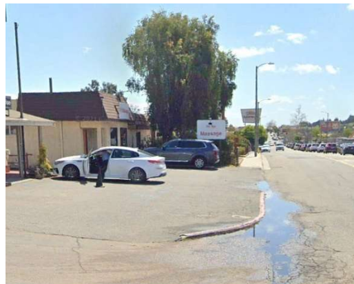
Figure 3: Parking lot extensions into sidewalk right of way
