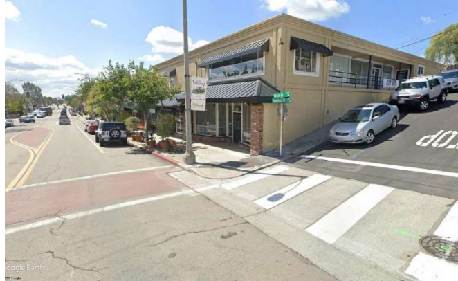
Figure 12: High Visibility Continental Crosswalk and Basic Crosswalk with Decorative Paving at Main Avenue and Hawthorn Street
