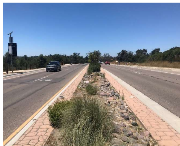
Figure 16: Example of a raised median
