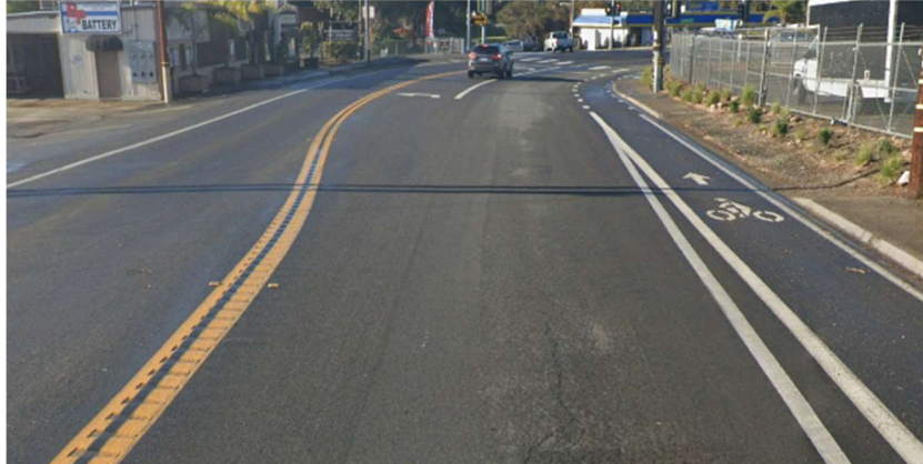
Figure 9: Existing Class II bike lane on East Mission Road east of Brandon Road
