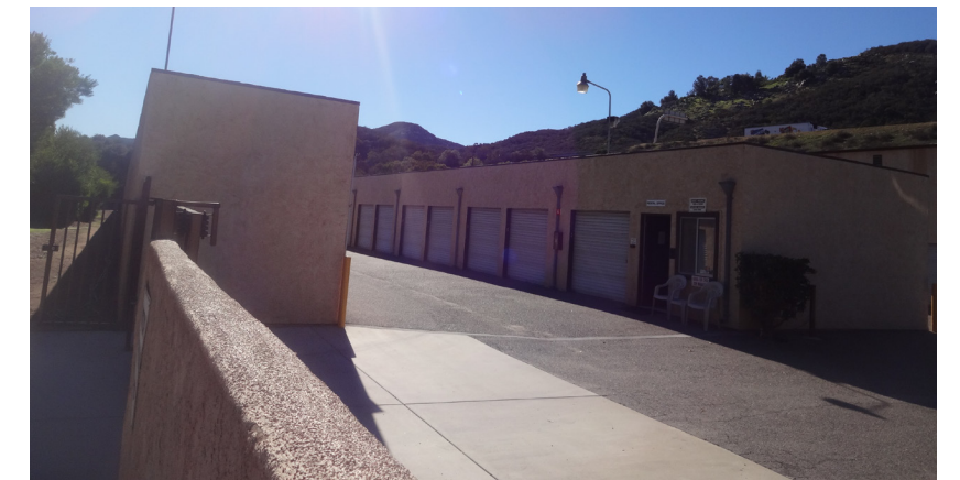
4 Facing south at the interior of the mini-storage complex within Sub-Area 7.
