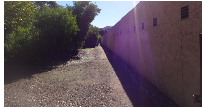
1 View along the front (eastern) façade of the mini storage complex on Sub-Area 7, facing south.
