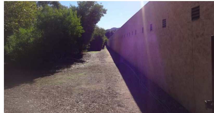
1 View along the front (eastern) façade of the mini storage complex on Sub-Area 7, facing south.
