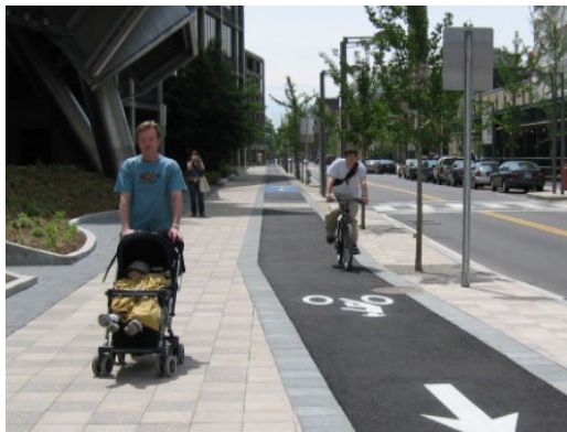
Photo 8: Example of Class IV separated bikeway adjacent to and at same grade as sidewalk (Cupertino, California)
