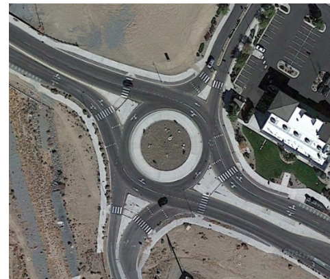
Photo 3: Typical two-lane roundabout with splitter islands (Sparks, Nevada)
