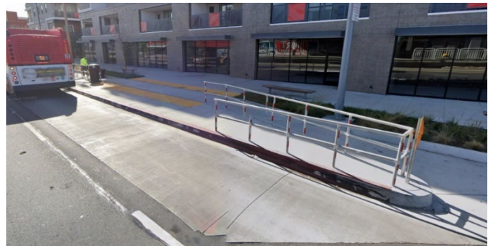
Photo 12: Example of sidewalk level crossing for pedestrians where bicycles ramp up and then down through bus stop. (Long Beach, California)
