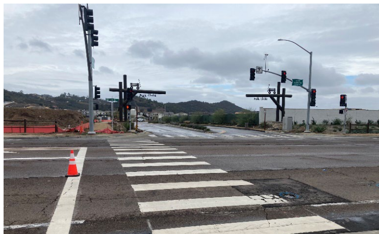
Photo 7: Continental crosswalk marking at Mirar de Valle Road along Valley Center Road.
