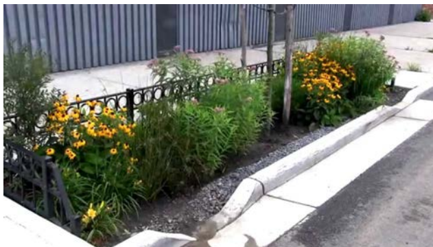
Photo 13: Bioswale incorporated into parkway to capture stormwater from the roadway. The dip in the curb allows the water to flow into the landscaped areas where the water then naturally filters through the soil and into the ground as opposed to flowing into storm drains.
