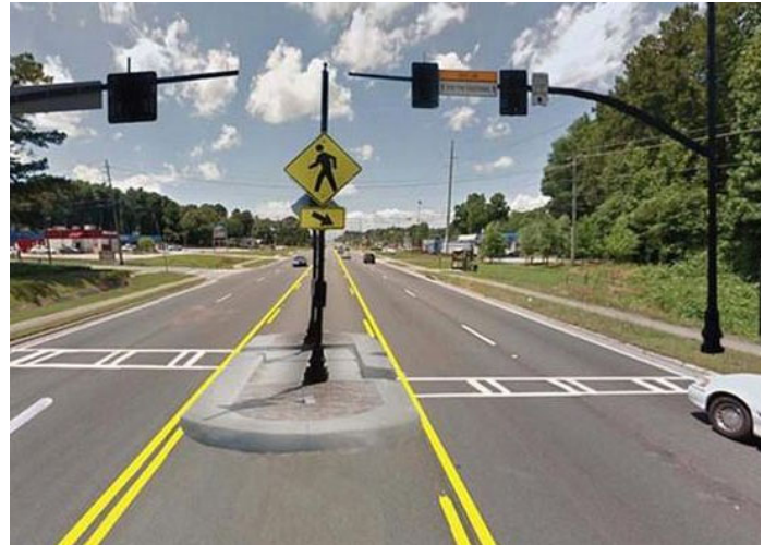
Photo 6: Example of signal-controlled crosswalk.
