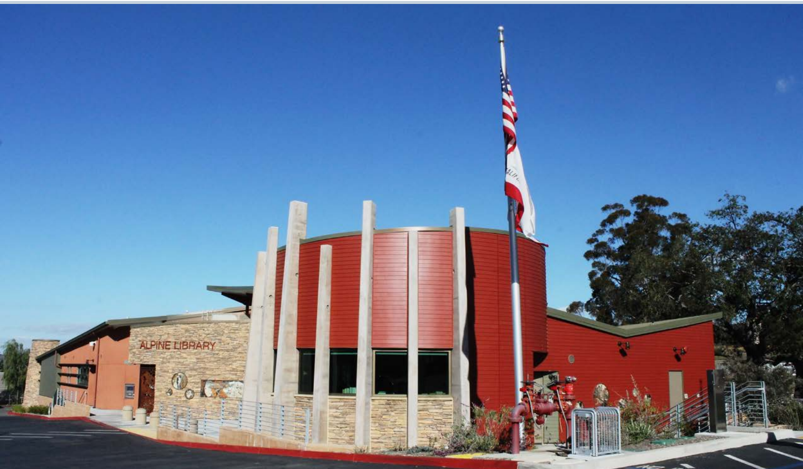
County staff uses building automation technology to track energy consumption and production at the zero-net energy Alpine Library.
