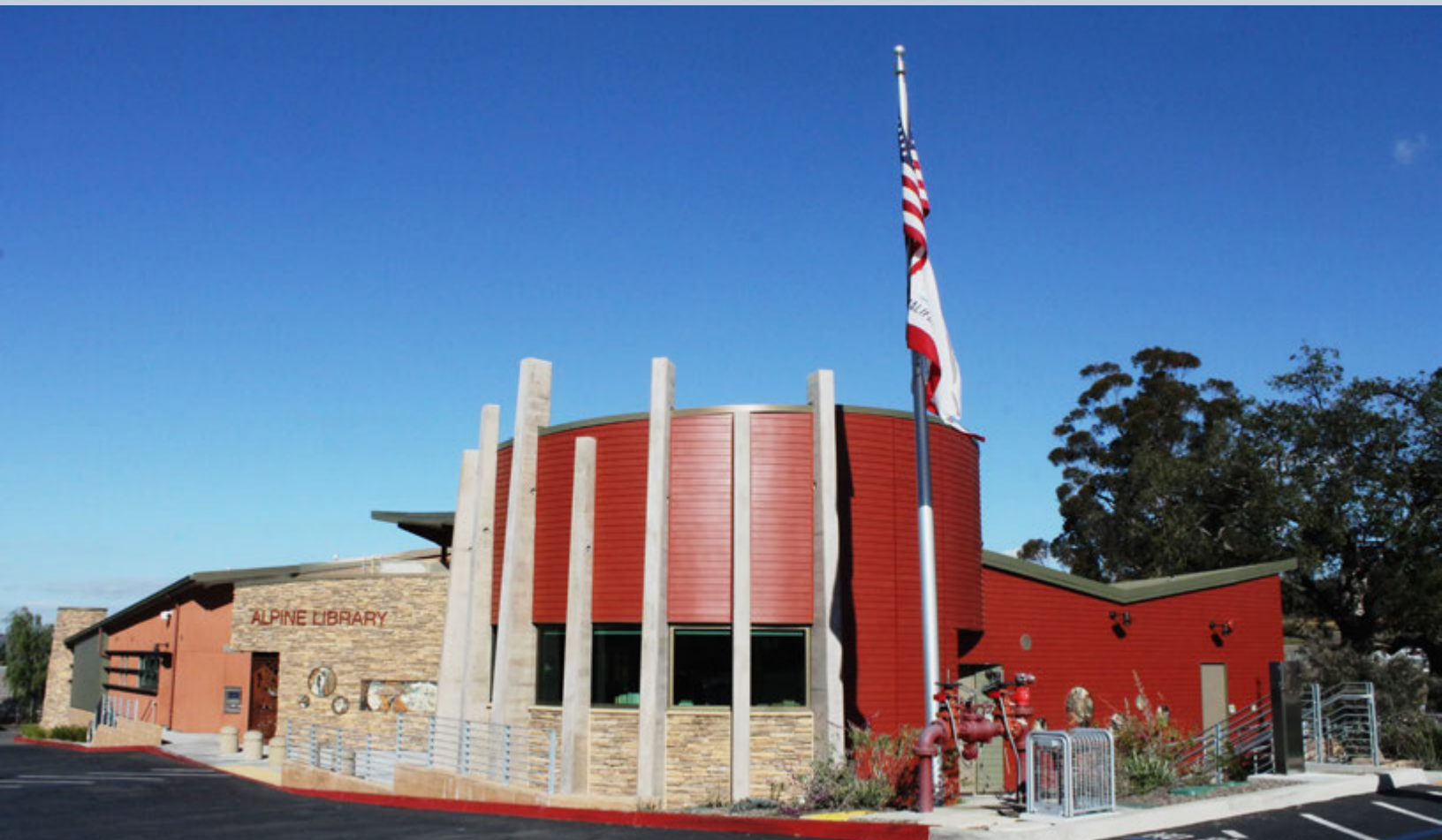
County staff uses building automation technology to track energy consumption and production at the zero-net energy Alpine Library.
