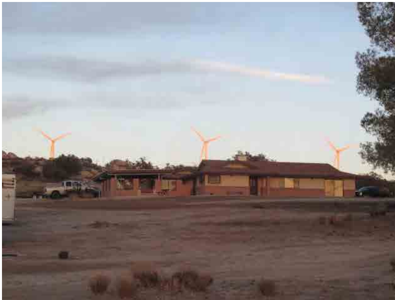
Figure 3 GE 2.3-107 ESS Wind Turbines at Tule Wind 4,300 Feet from Guy Residence
