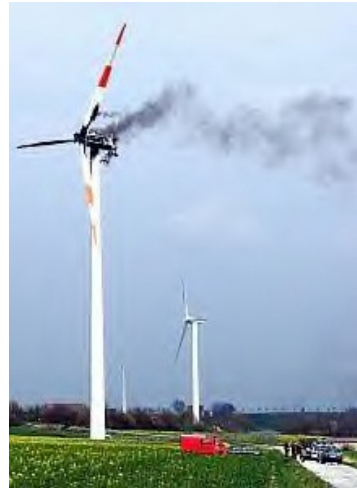
Figure E.6.1: Turbine fire in east Germany. Fire brigade has cordoned off the area to allow the fire to burn out.
