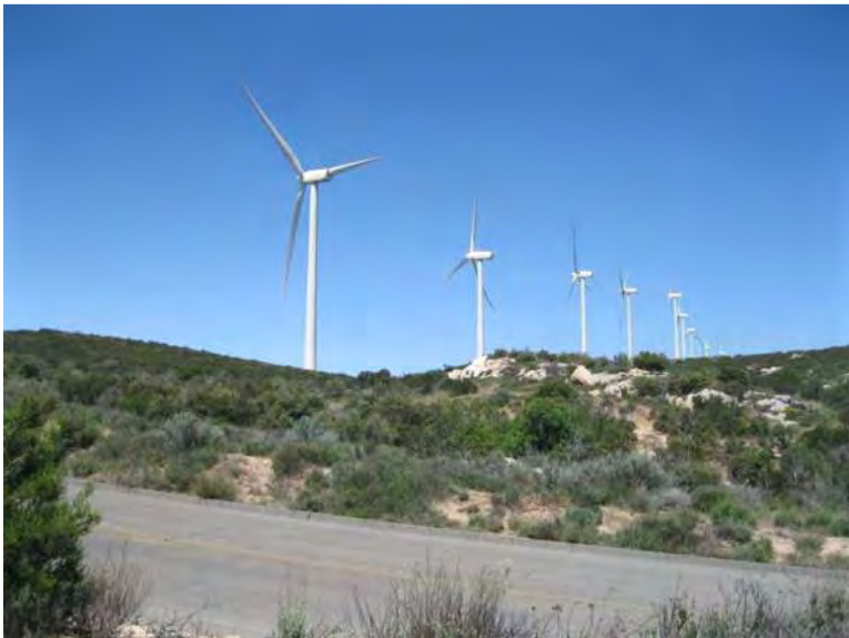
Figure 1 Wind Turbines at Kumeyaay Wind
