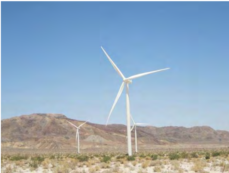
Figure 2 Wind Turbines at Ocotillo Wind
