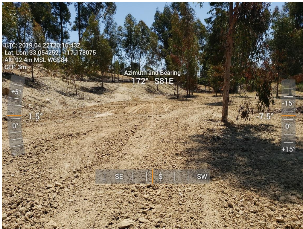
Photograph 1. View from lower pad area looking south.
