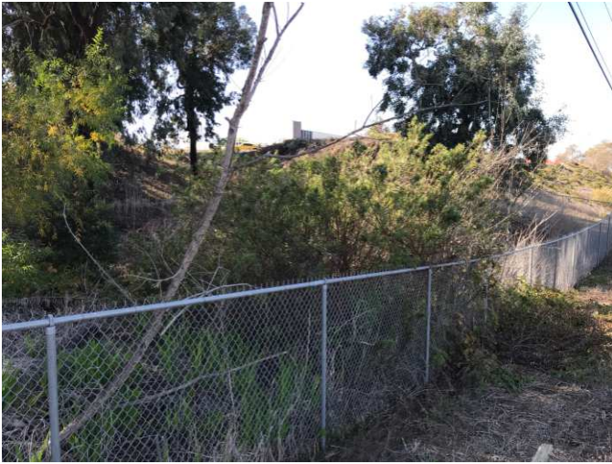
Photograph 1: View of the southern end of Drainage Feature 1, facing west.
