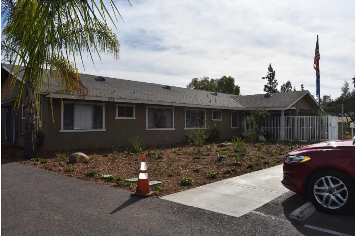
Photograph 8 West Elevation of Building 1, View Southeast
