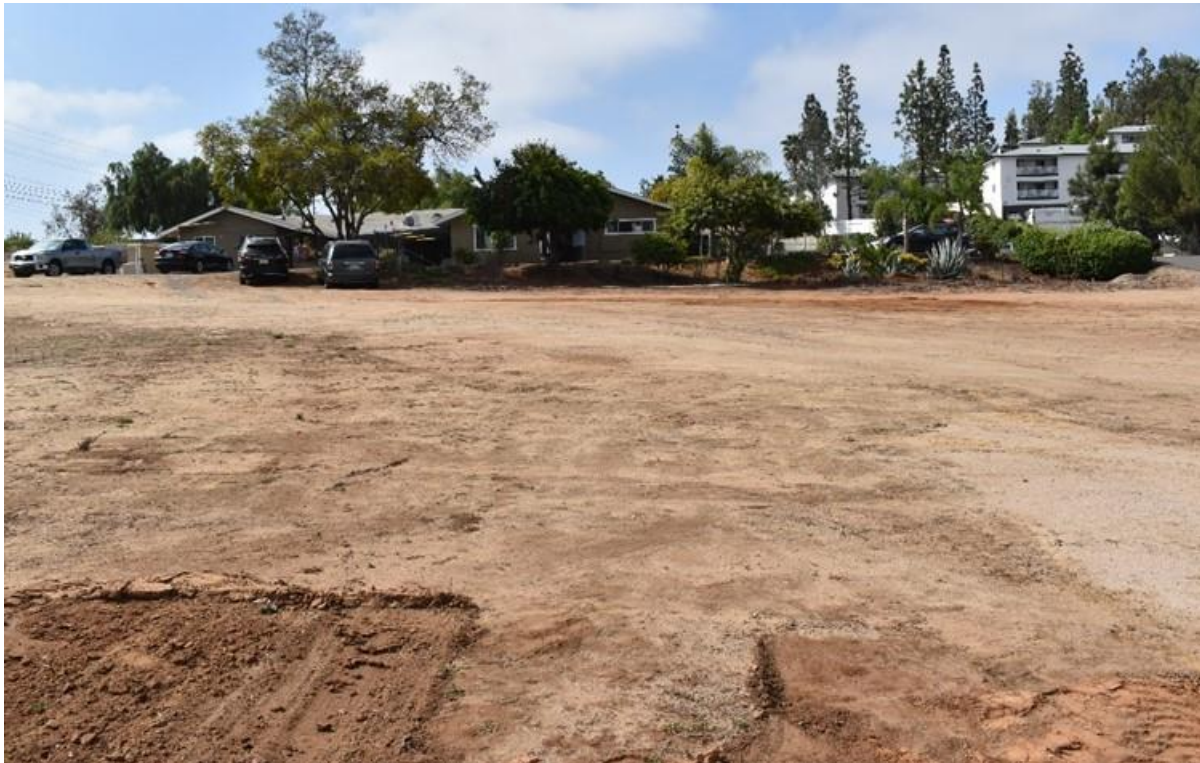
Photograph 3 Building 1, View South
