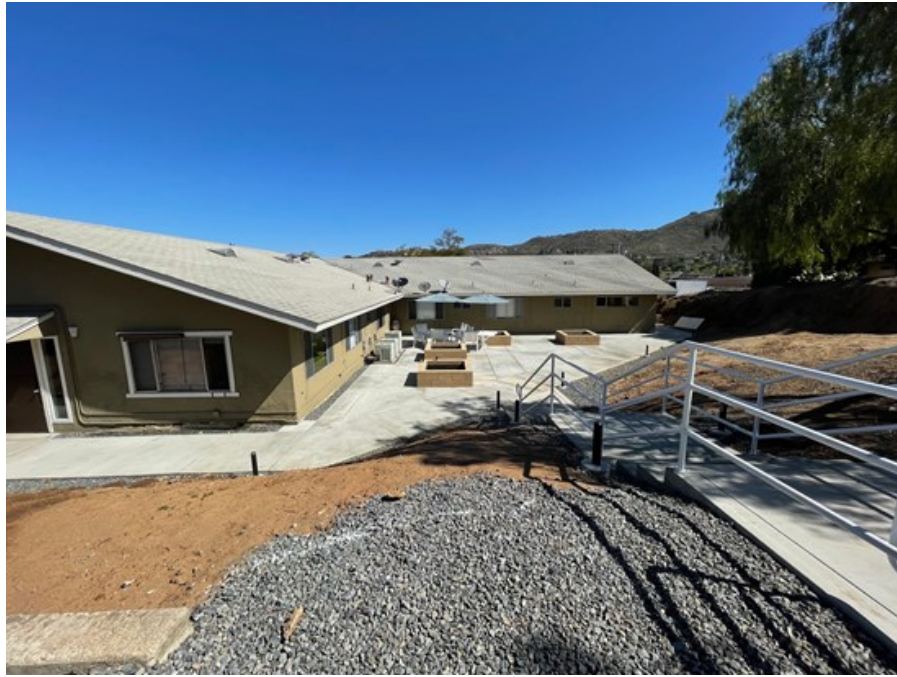
7. Looking north towards south side of Building 1.
