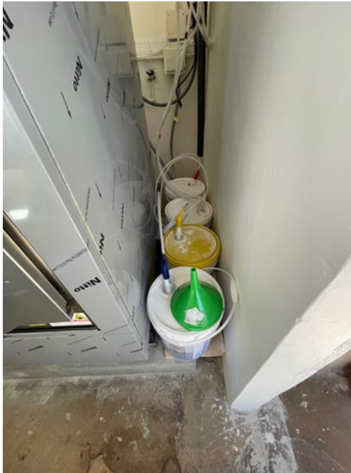
23. Laundry supplies in laundry room on east side of Building 1.
