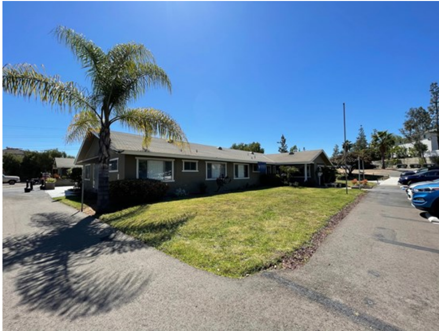
1. Looking southeast towards Building 1.
