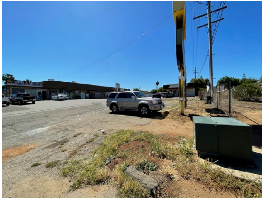
31. Adjoining property to the east. Note transformer and former groundwater monitoring well and remediation piping locations.
