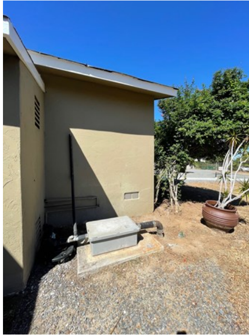
11. Grease trap near north side of western portion of Building 2.
