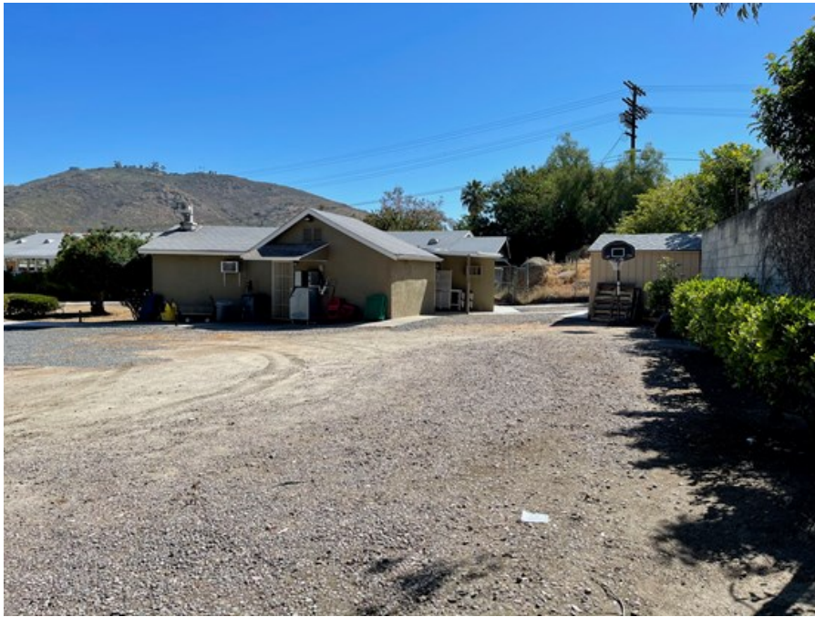
9. Looking east along north side of subject site, towards Building 2.
