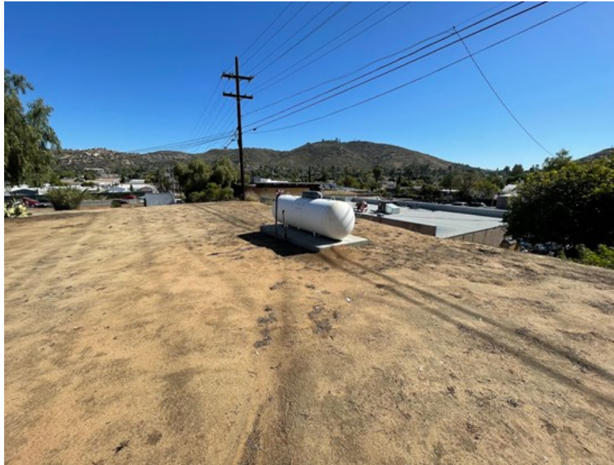
13. Propane tank for emergency generator, east side of subject site.
