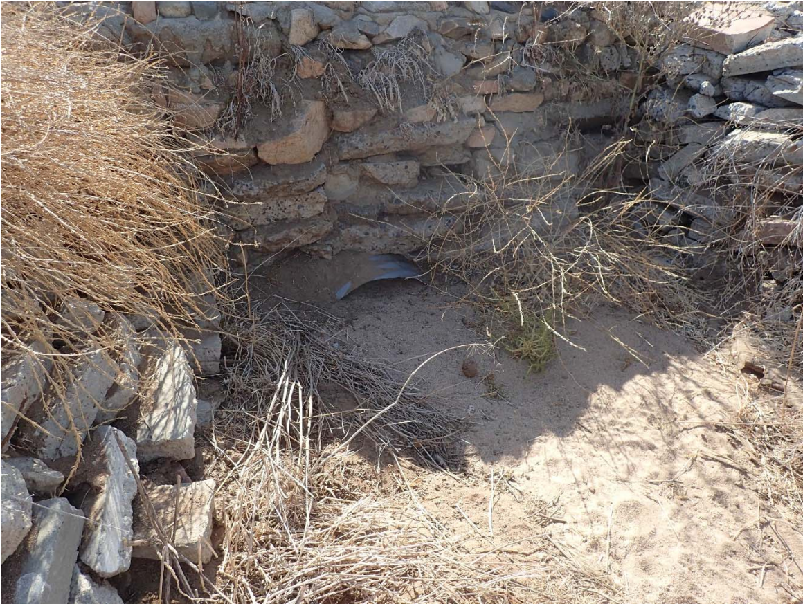
Figure 5. Roadway Culvert at Lower End of Reach 3H
