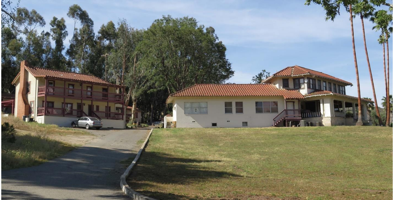
Photo 6: View of Historic Residential Structures
