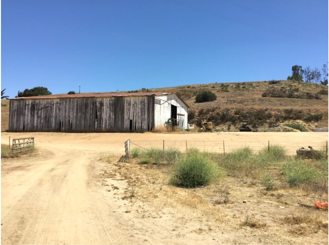
Photo 4: View of Existing Barn
