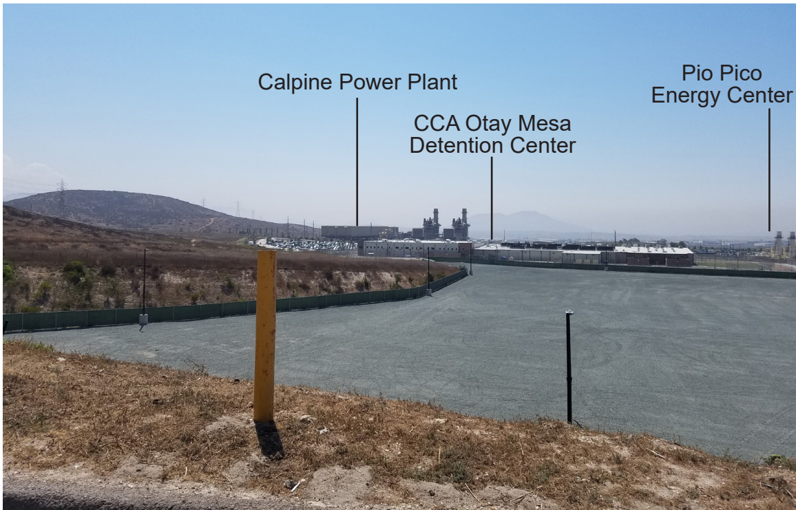
View 3: View southward toward construction/grading in Project vicinity from parking access road to lot of Alta Cafe (old Kuebler Ranch). (2017)
