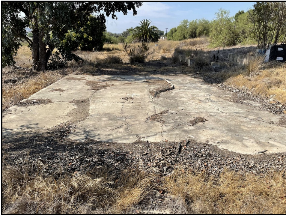
PHOTOGRAPH 3 Overview of Foundation #2, Looking Southeast
