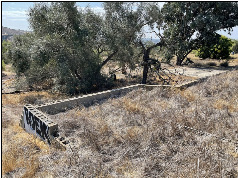
PHOTOGRAPH 2 Overview of Foundation #2 Area, Looking Southeast
