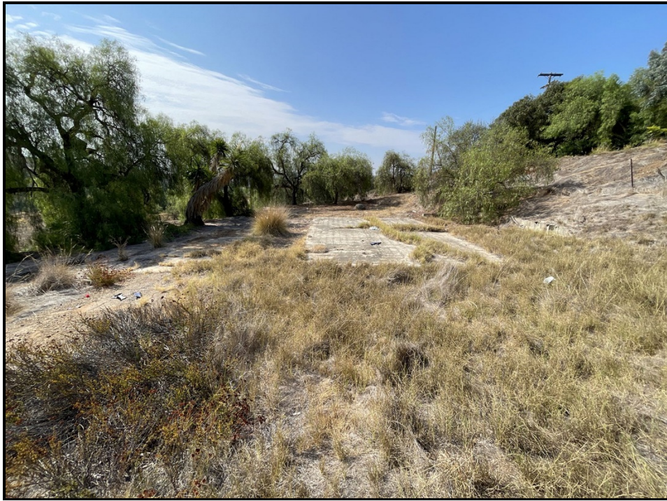
PHOTOGRAPH 1 Overview of Foundation #1, Looking South
