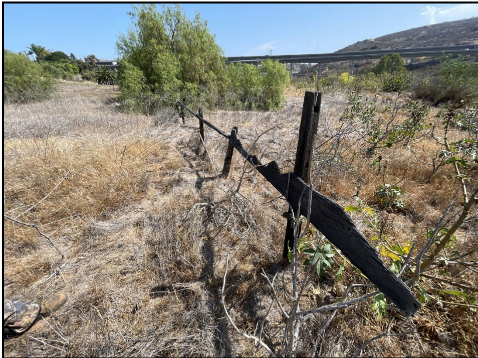
PHOTOGRAPH 6 Overview of North-South Fence Portion, Looking North
