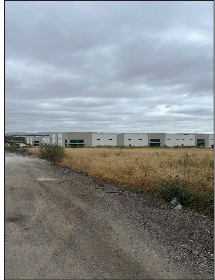
Photograph 2. View facing southwest towards the western portion of the project site standing along Harvest Road. Note the newly constructed warehouse structure located south/southwest of the proposed project.
