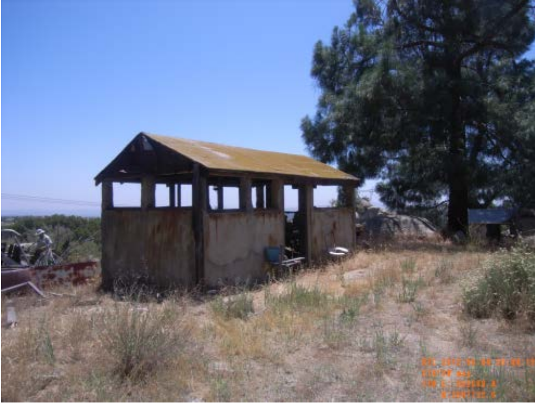
Figure 4.10 Overview of the ancillary (kitchen) structure at CA-SDI-7000
