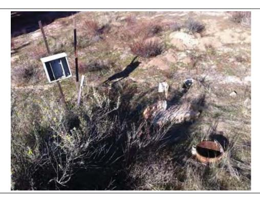
Photograph 15. Steel casing for a water well (lower right) located on the SE part of the subject property
