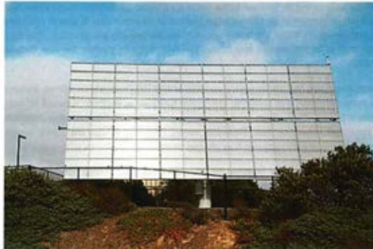
Fig. 51 Glare due to Soitec Solar installation on a typical day [Photo taken at the campus of the University of California San Diego at 5:00 pm, on September 20, 2013].
