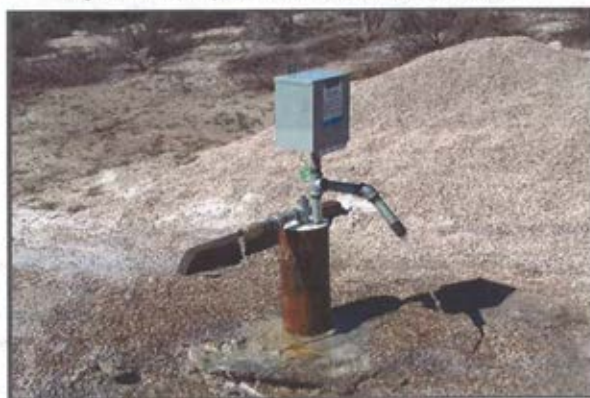
Fig. 48 New water well near Walker Creek, flowing under artesian conditions on September 18, 2013.
