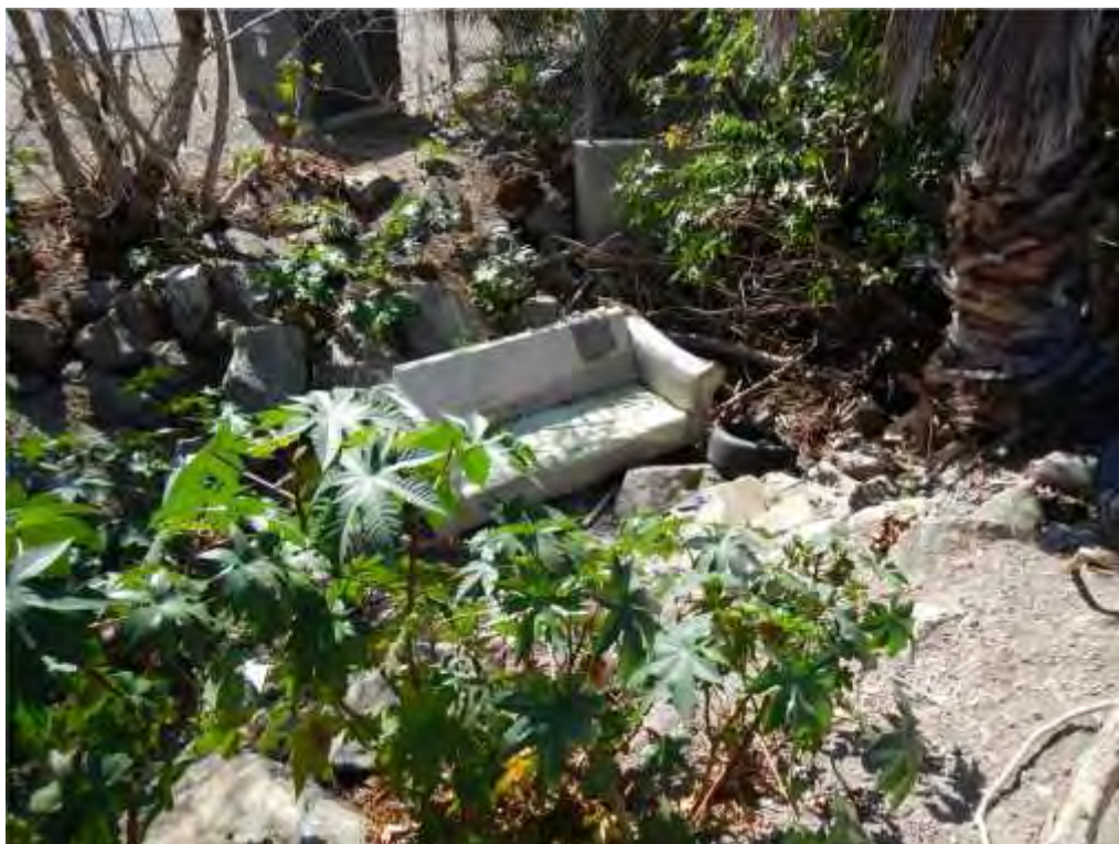
Photograph 16 – End of Drainage 1 looking downstream/southwest near southern border of project site. Concrete culvert outlet visible in background.
