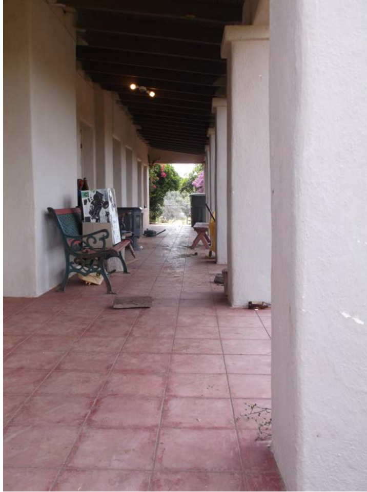
Figure 9. Arcade at southwest façade, facing east-southeast.
