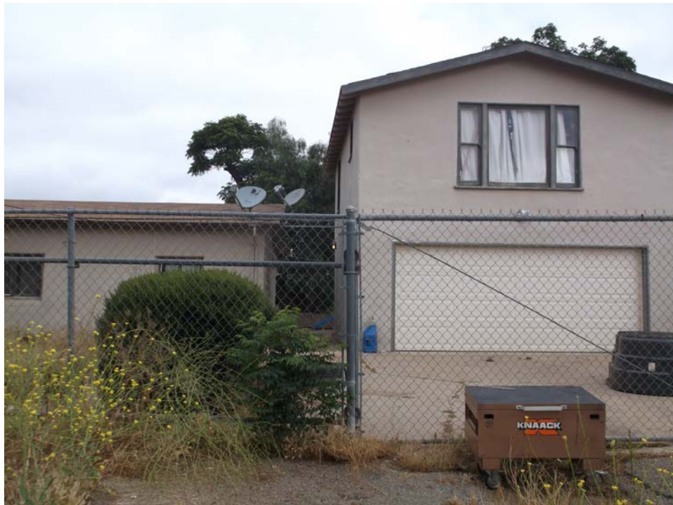
Figure 10. Southeast facades of residence's ell wing and garage, facing northwest.
