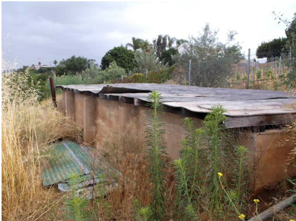
Figure 5. Concrete cistern, facing north-northeast.
