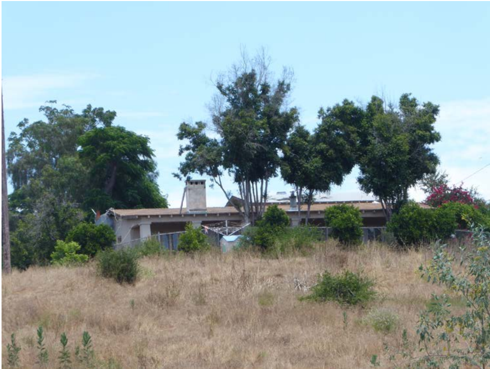
Figure 7. Residence and surrounding landscape, facing northeast.
