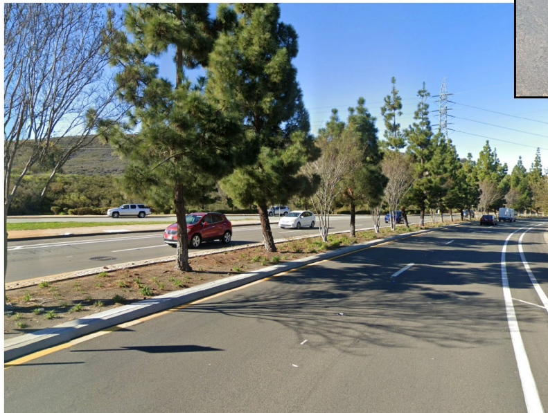
View 2 - East of the Project Site looking Northwest.
