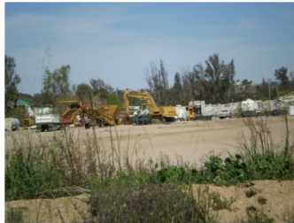
Facing north at equipment storage
