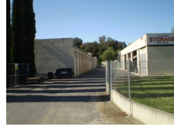
Facing south at storage units
