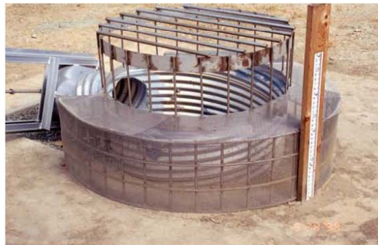
Figure 1 Example of Extended Detention Outlet Structure
