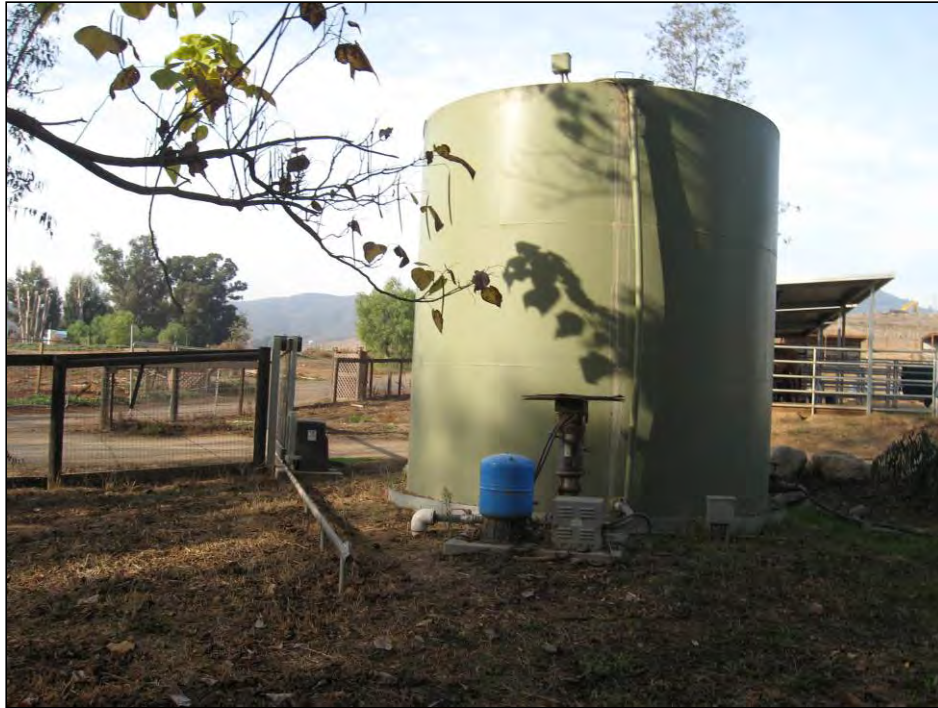
Photograph #13 2,000-gallon irrigation water AST on the southern portion of the Site.
