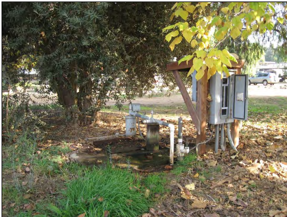
Photograph #12 Irrigation groundwater supply well on the southern portion of the Site.
