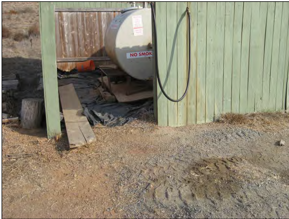
Photograph #14 200-gallon diesel AST in the south-central portion of the Site.
