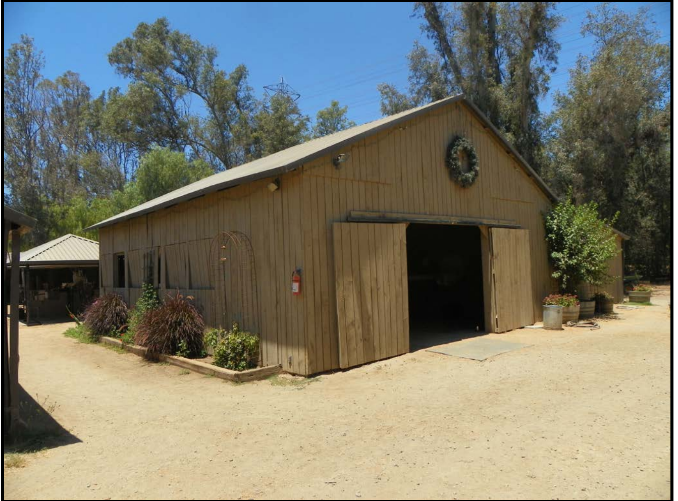
Figure 22: Barn south side.
