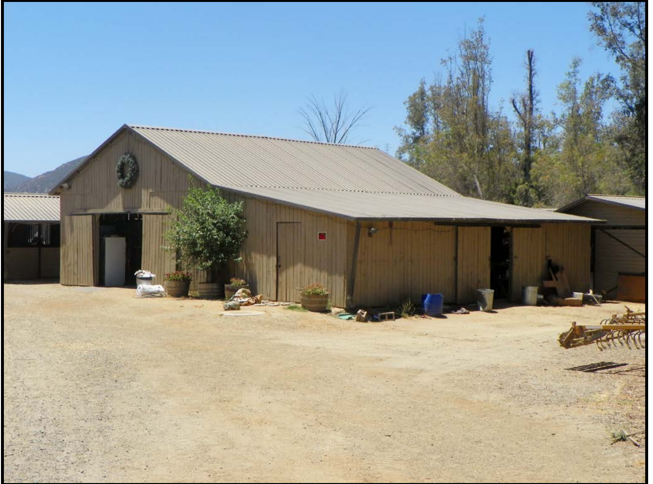
Figure 21: Barn, north side.
