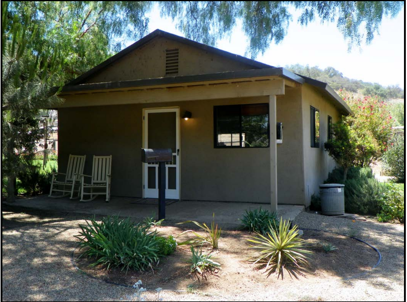
Figure 14: Building B front (north) side.
