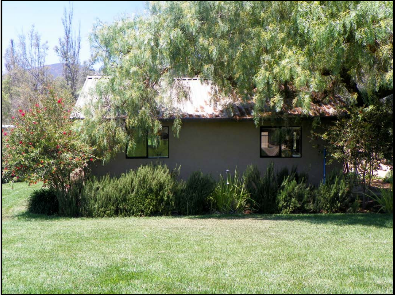
Figure 16: Building B, north side.
