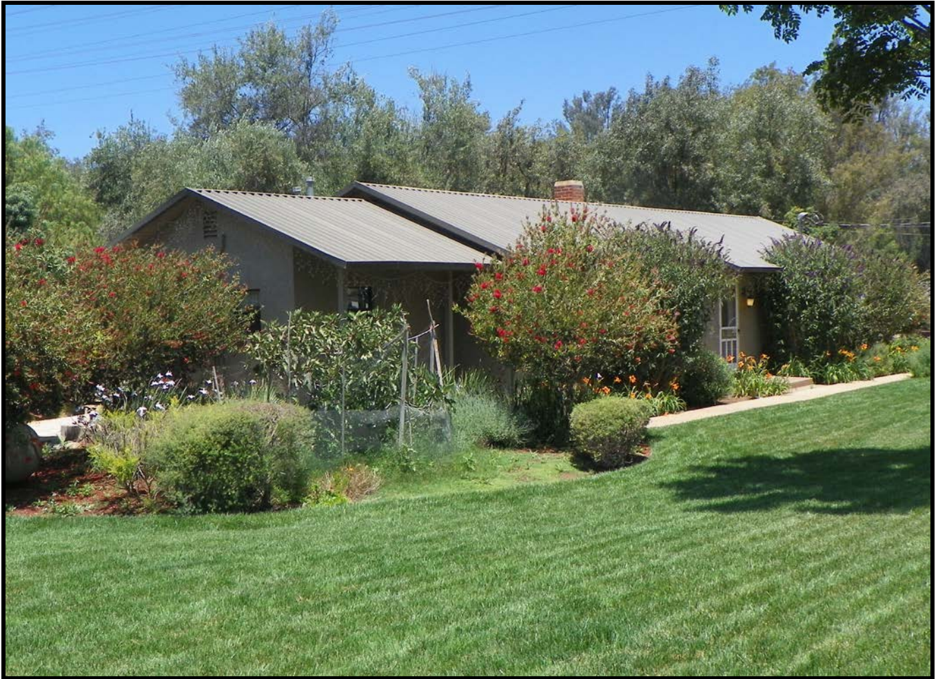
Figure 13: Building A, west end.
