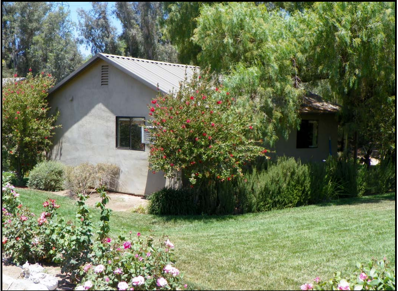
Figure 15: Building B, back (south) side.
