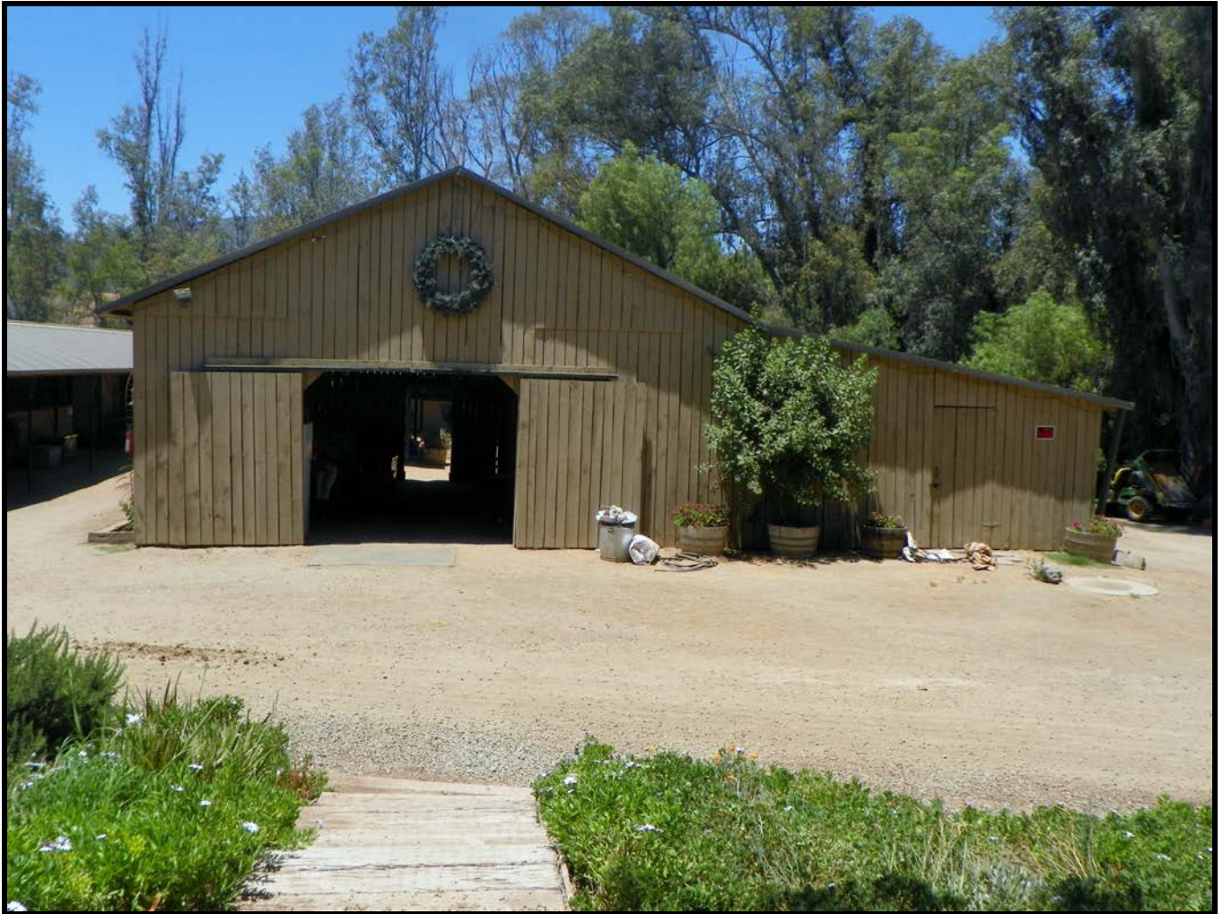
Figure 20: Barn Structure C, front (east) side.
