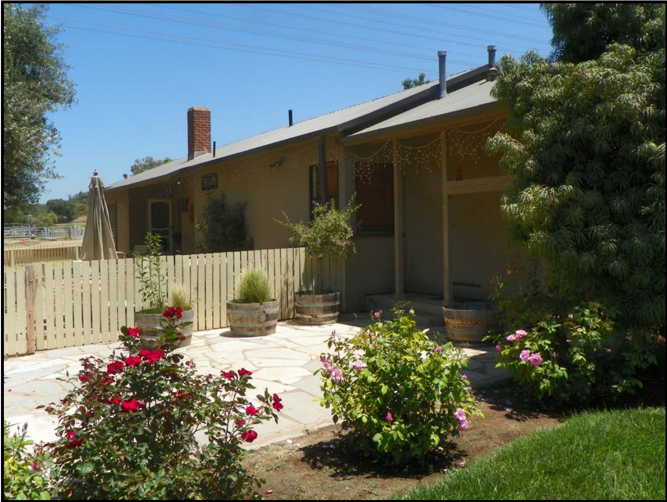
Figure 12: Building A, back (west) side.
