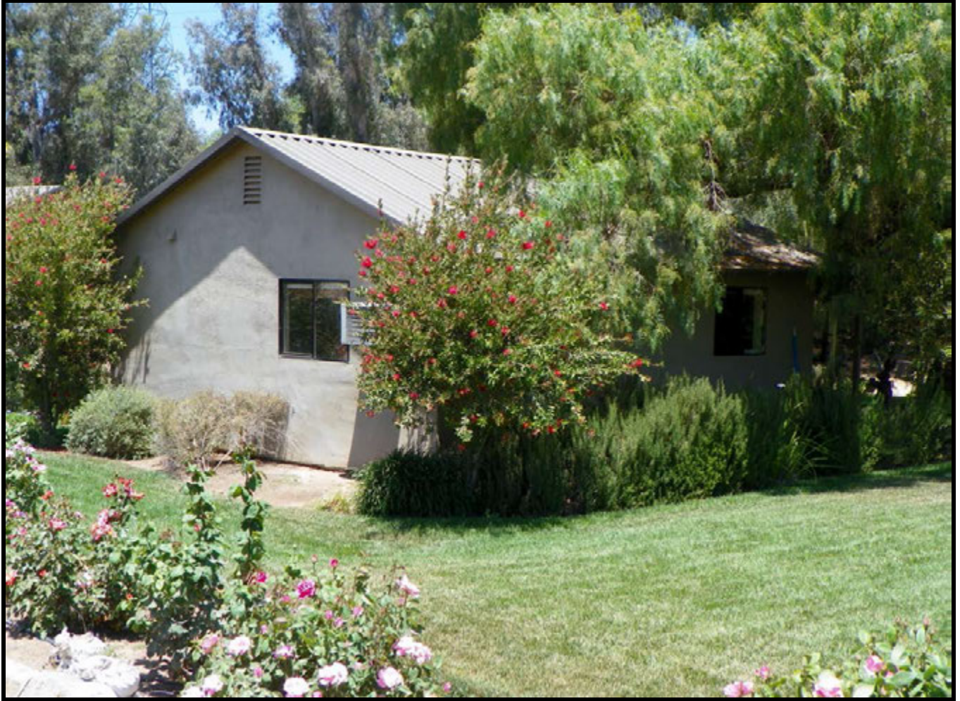
Figure 15: Building B, back (south) side.
