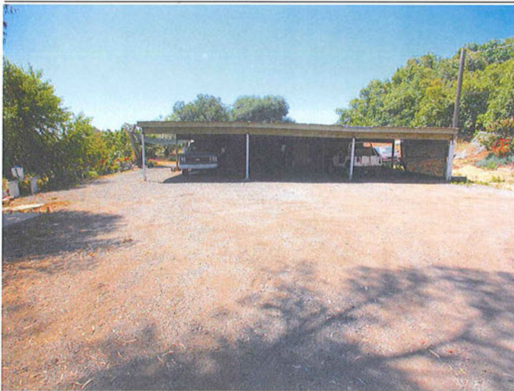
Plate 6.6-3 View of the north end of the equipment shed, facing south.
