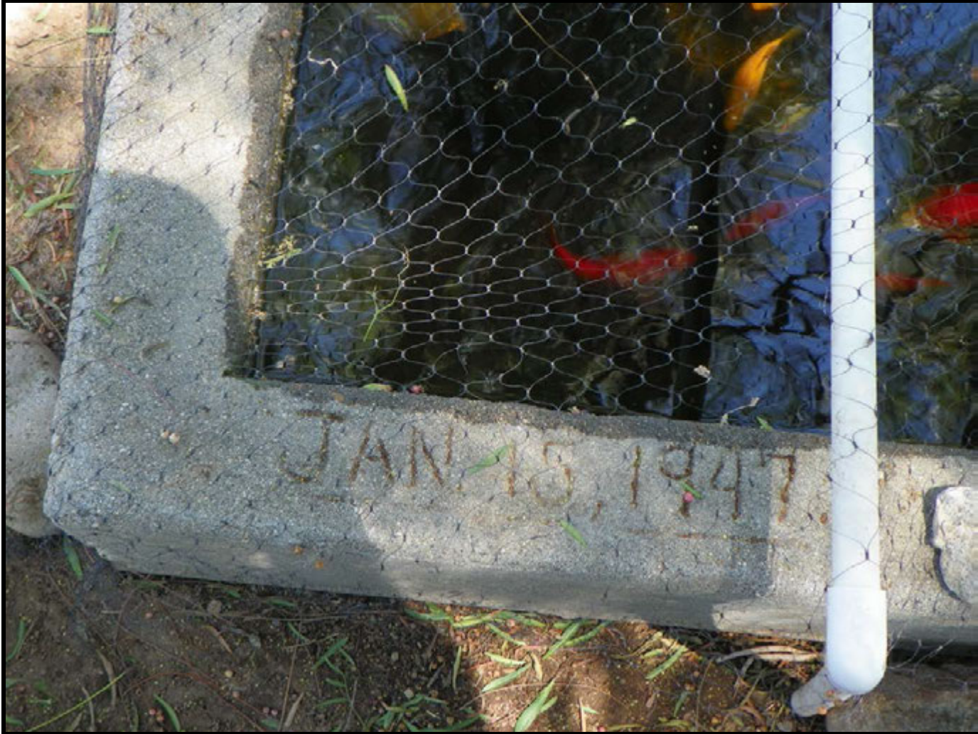
Figure 18: Date inscribed in concrete at southwest corner of fishpond.
