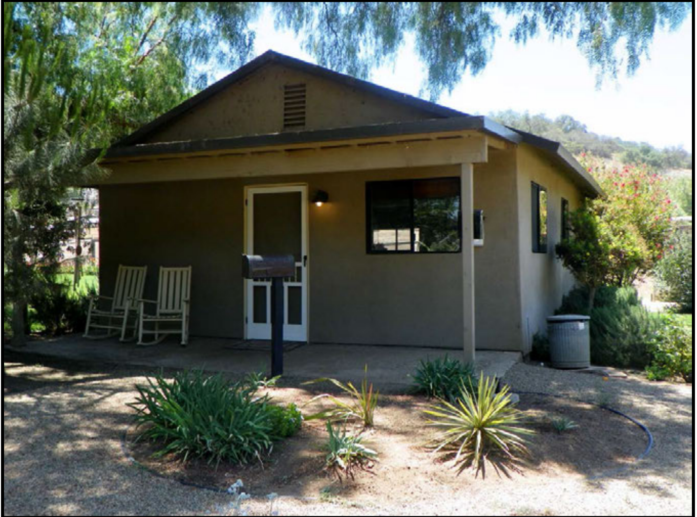
Figure 14: Building B front (north) side.
