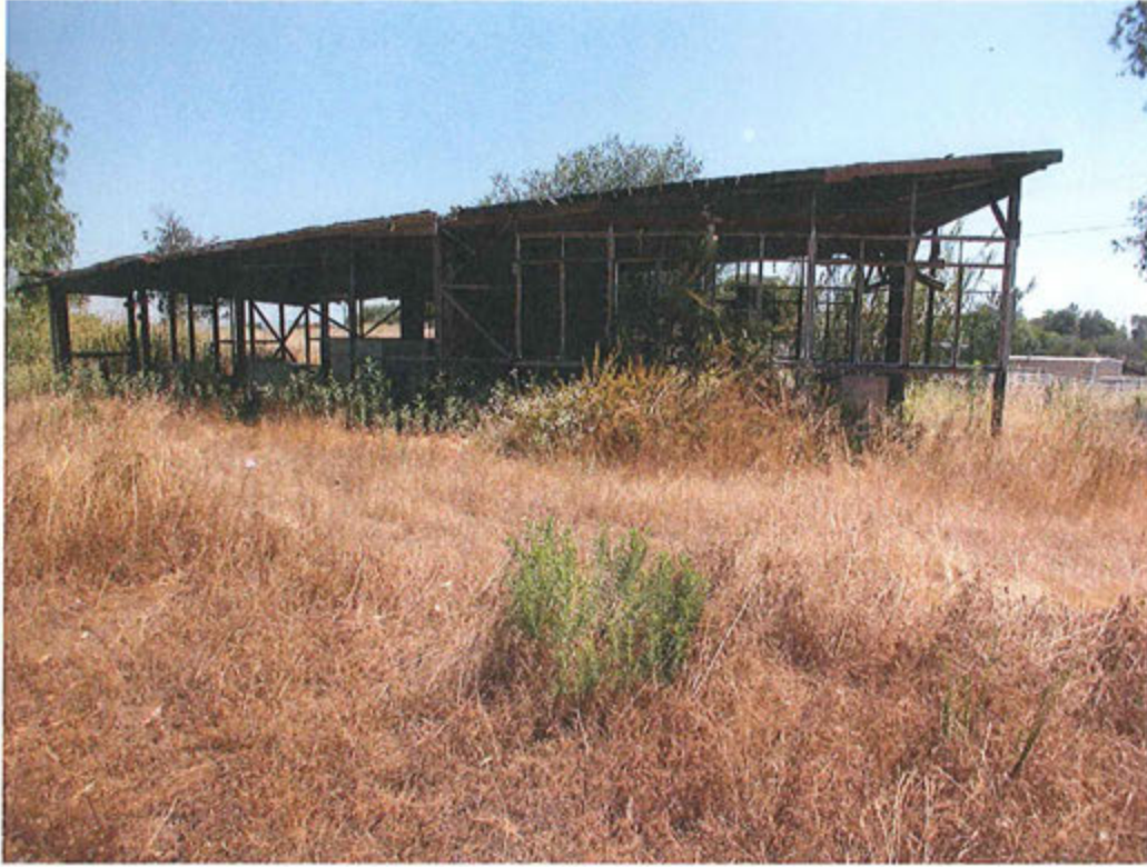
Plate 6.6-6 View of the west side of the pump house, facing east.
