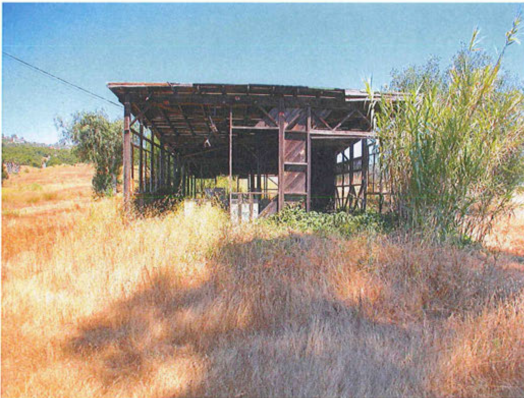
Plate 6.6-7 View of the south side of the pump house, facing north.
