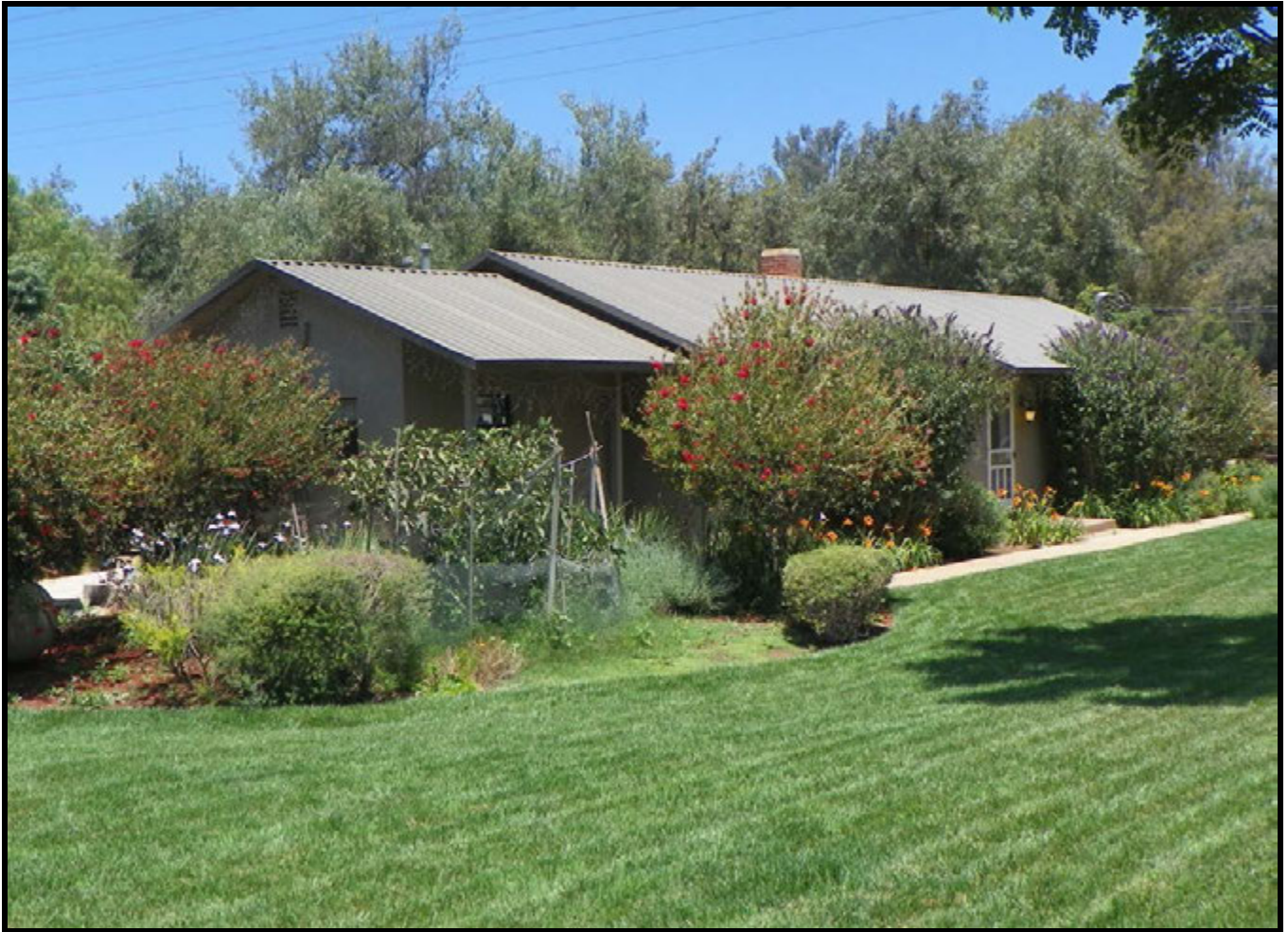
Figure 13: Building A, west end.
