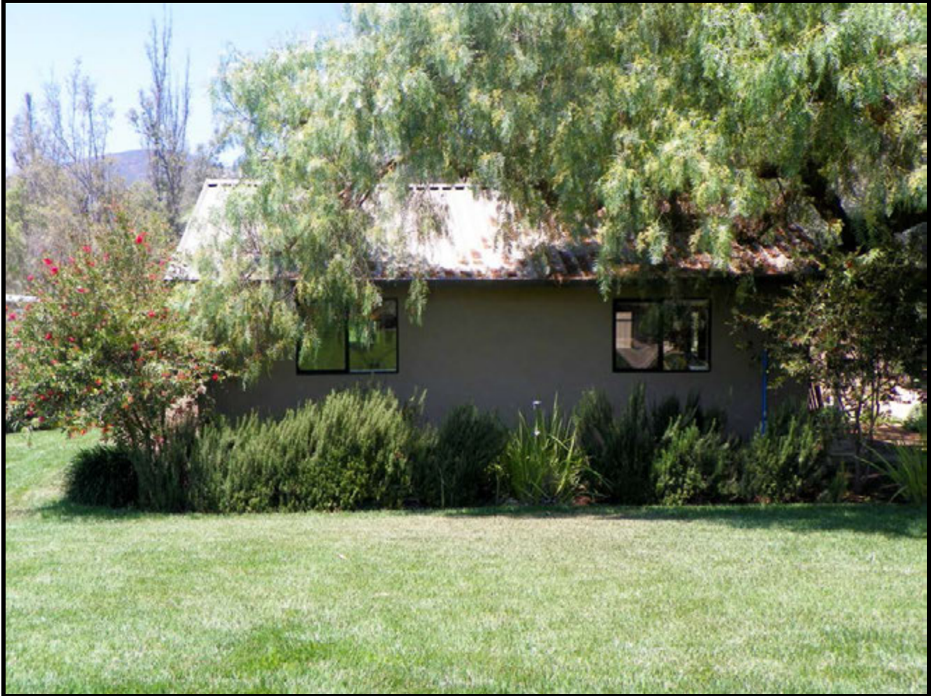
Figure 16: Building B, north side.
