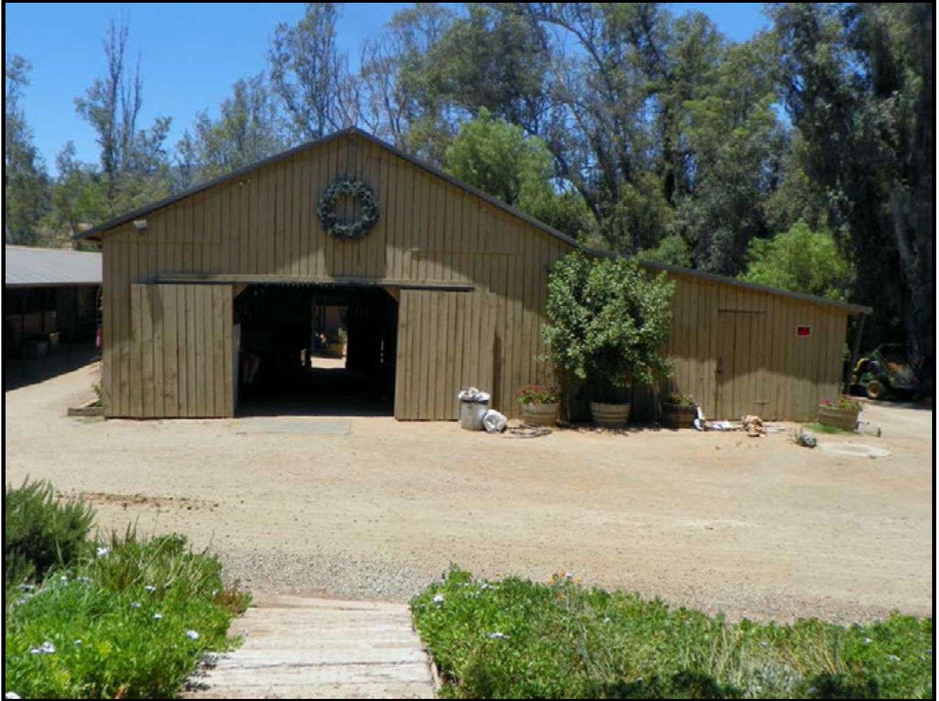
Figure 20: Barn Structure C, front (east) side.
