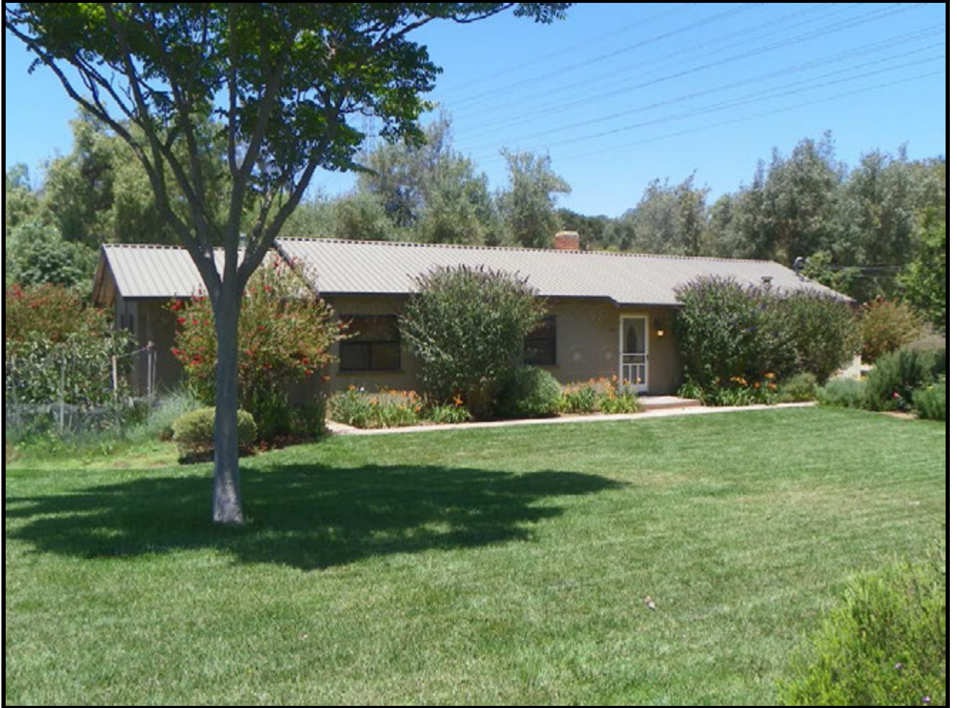
Figure 11: Building A, front (east) side.
