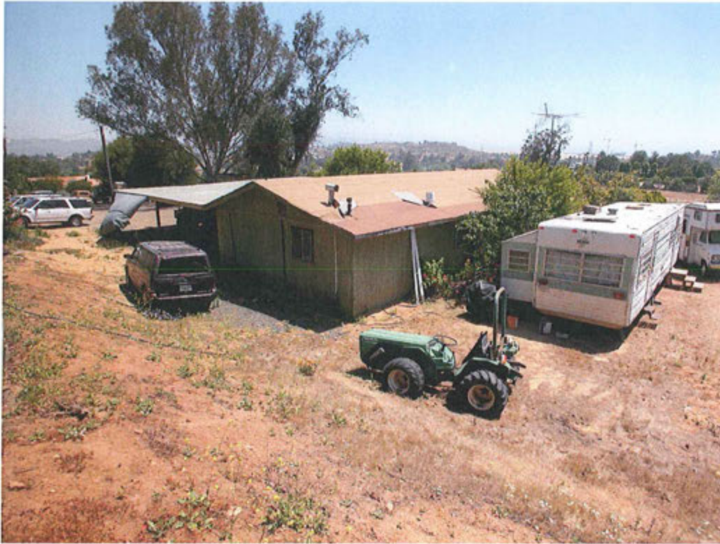
Plate 6.6-2 View of southwest corner of foreman's house/shed, facing northeast.
