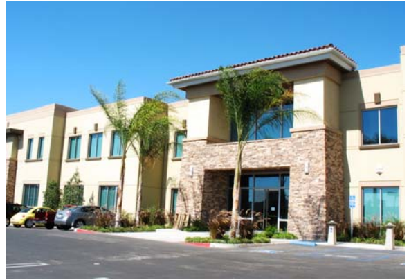
Office complex in Rancho San Diego
