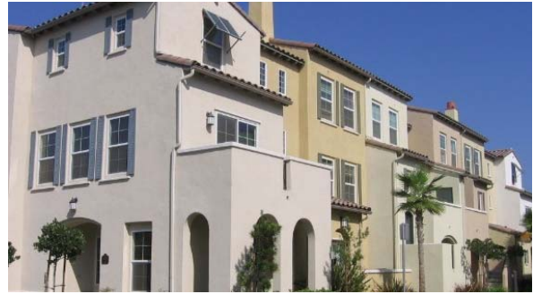
Multifamily housing in 4S Ranch
