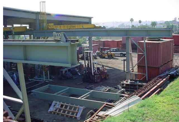
Steel fabricating plant in Spring Valley
