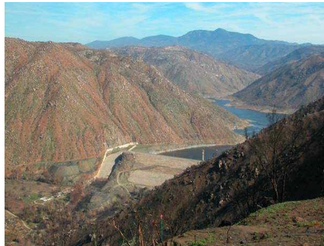
Dam in unincorporated County
