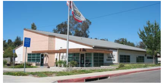
Fallbrook Sheriff substation
