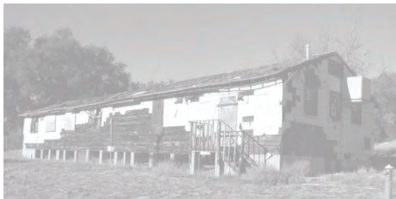
Camp Lockett WWII Supply Building
