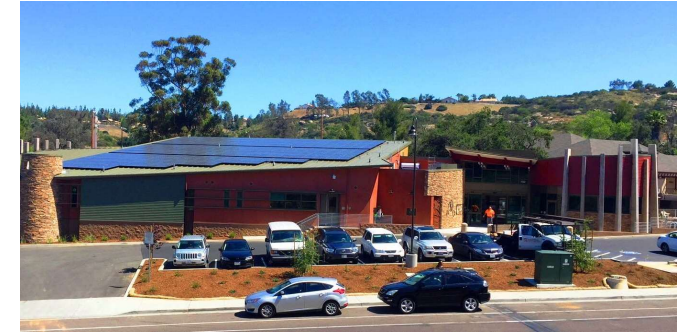
The Alpine Branch Library is a zero net energy facility
