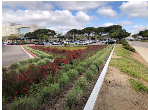
Drainage swale at the North County Regional Center in Vista
