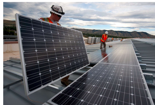
Worker installing rooftop solar panels
